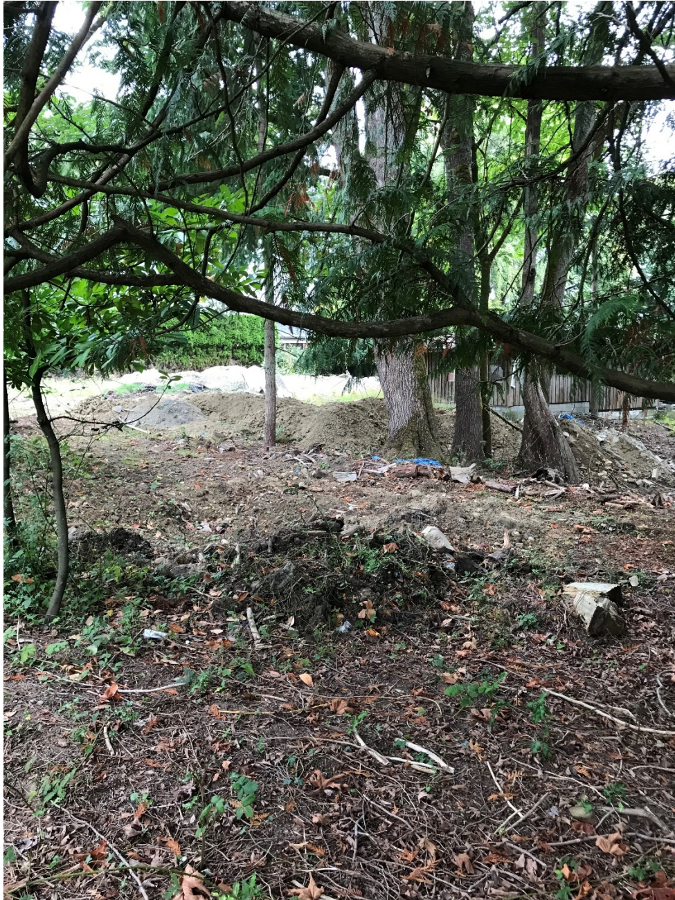
Exhibit 4-B: Grading within drip lines of trees; Debris in soil. Photo taken 10/07/2020.
