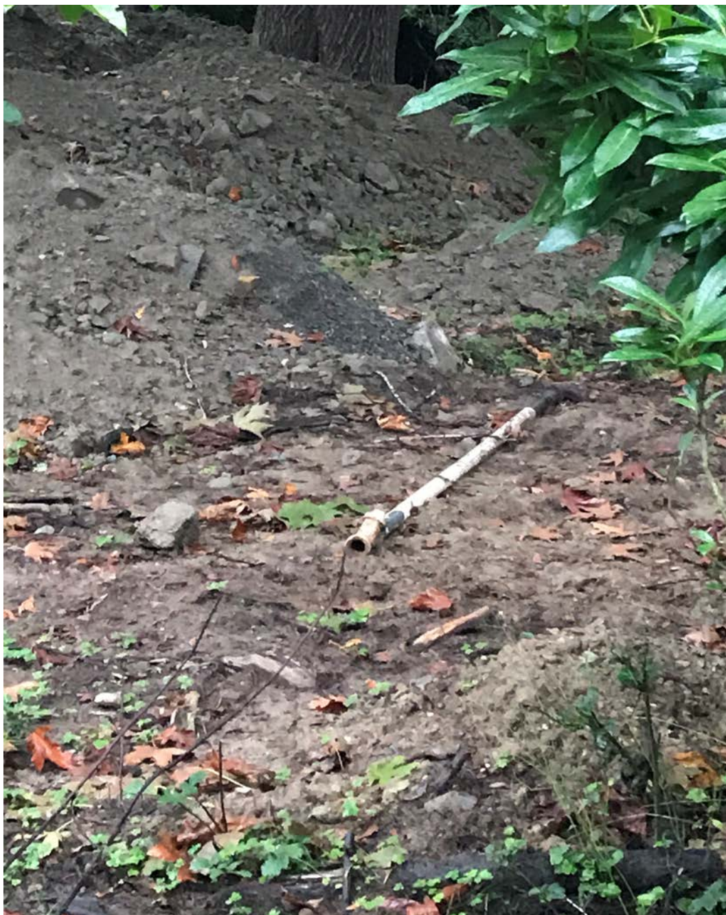
Exhibit 4-D: Construction Debris Photo taken 10/19/2020.
