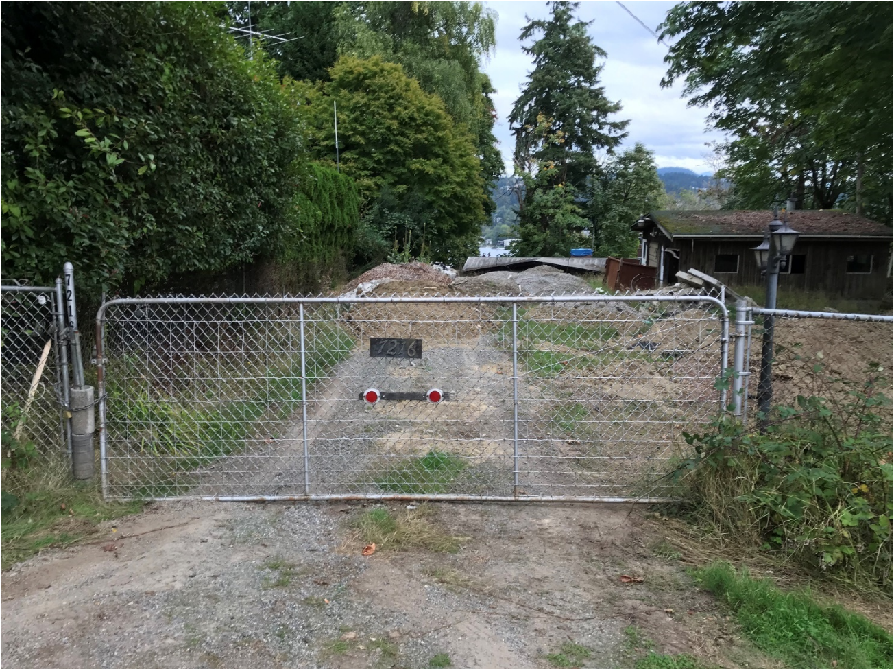
Exhibit C: Stop work order removed; Additional grading. Photo taken 10/09/2020.
